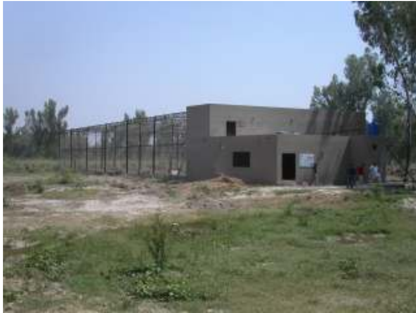
Figure 4 the service building attached to the holding aviary
